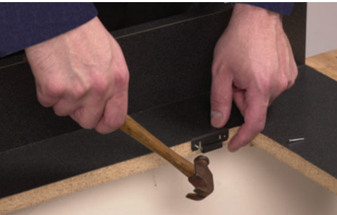
1 Nail Spring clips to the edge of the counter top
