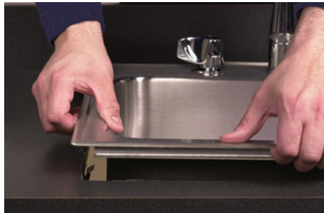
2 Apply caulk to underside of the bowls rim
